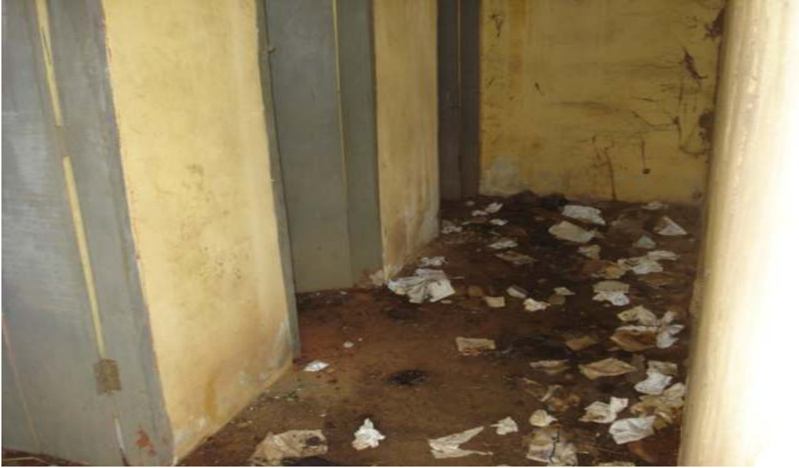
Entrance into a typical public school toilet
