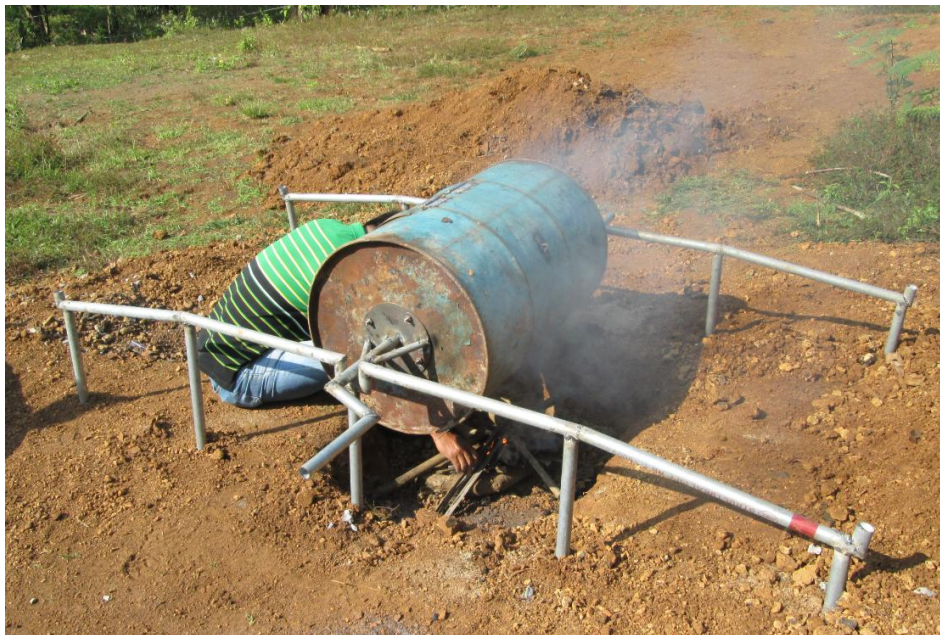
Figure 3: Spent two days building this Biochar drying pit and this is the pit in action!
