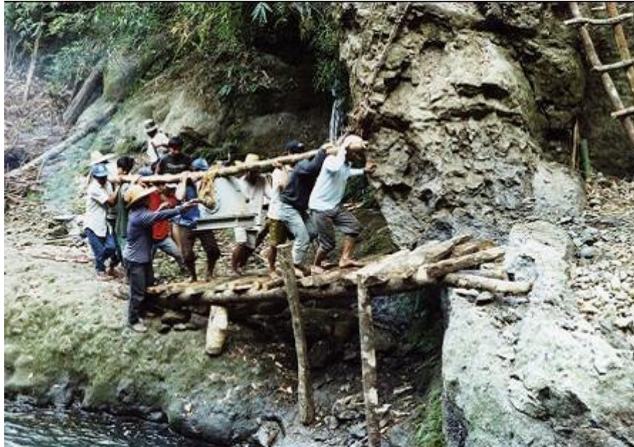
Figure 61. Hauling the turbine to the powerhouse site
