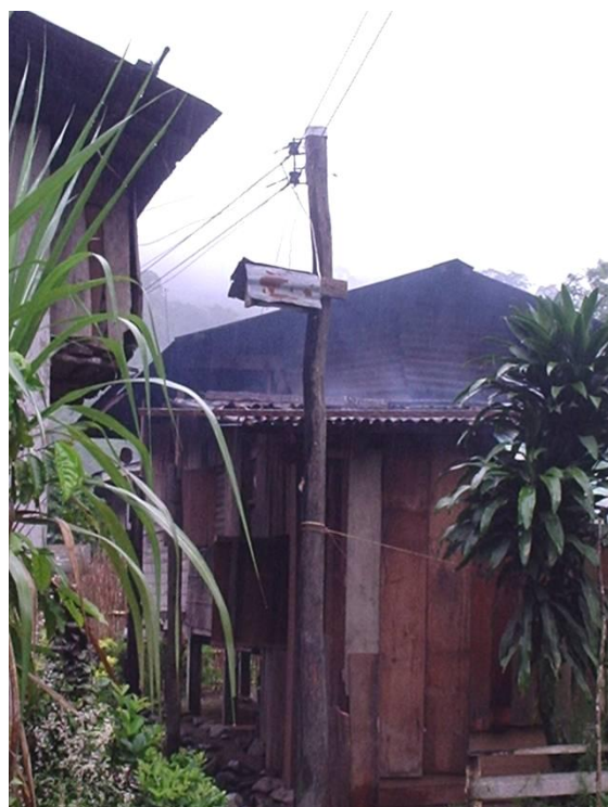
Figure 34. Wooden Transmission post of Buneg MHP
