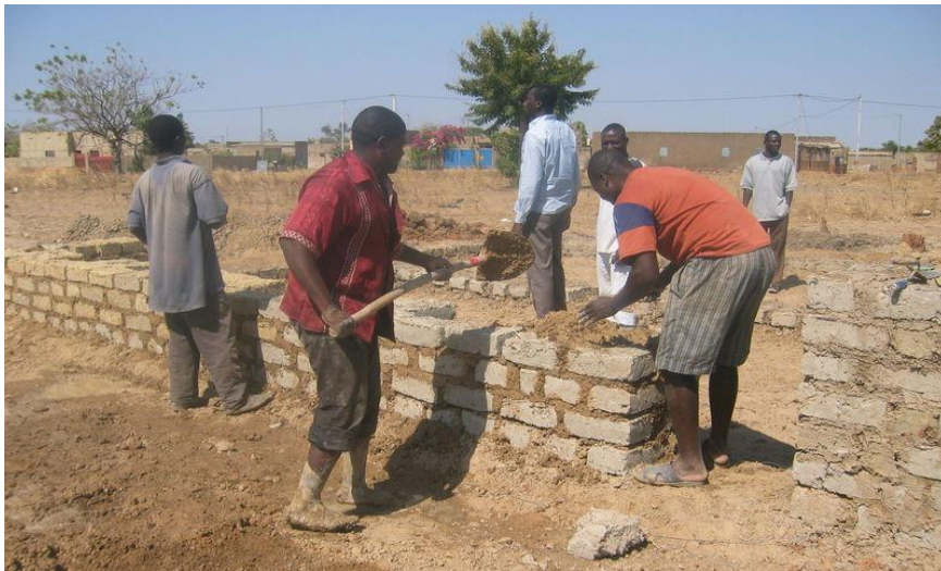
The two first Zambian AVN apprentices in the programme, Jaspas Moobela and Christopher Phiri (foreground), working on construction of a school library in Boromo, Burkina Faso (Jan, 2010)
