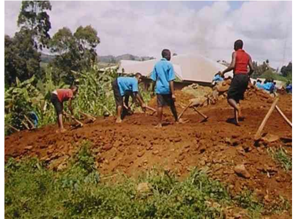
Students doing ground work at the plot
