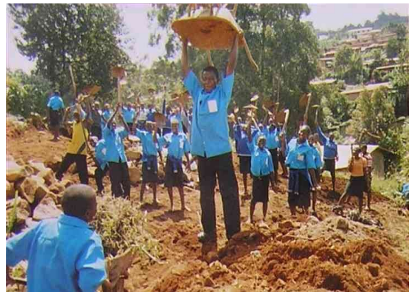
Excavation at the plot
