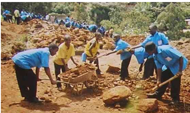
Students preparing the plot for the laying of the Foundation
