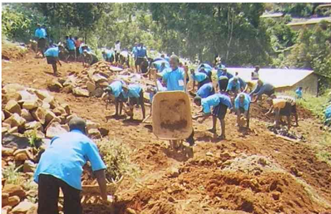
Excavation at the plot
