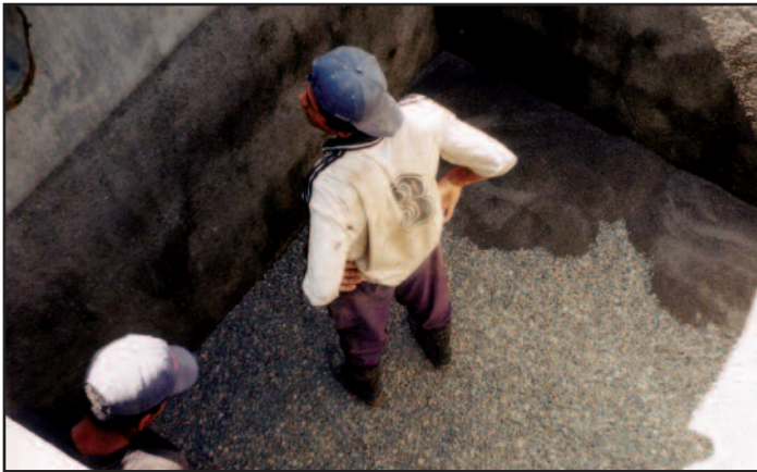
The village water committee completes the loading of the slow sand filter 1-cm stone and then fine sand.
