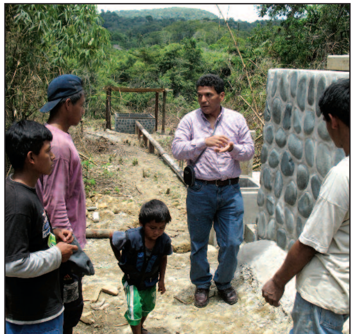
HOTC Sanitary Engineer Moises Mera, supervises the construction of the septic system. This system naturally decomposes waste without chemicals or handling of the waste. The end result fertilizer.
