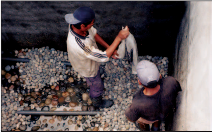
The village water committee loads the slow sand filter serving the central community. This is the first layer of 10-cm rock.
