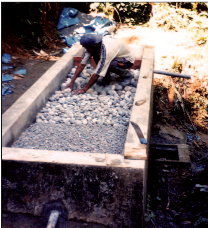
A village water committee member puts the finishing touches on the roughing filter comprised of 10-cm, 5-cm, and 1-cm stones.
