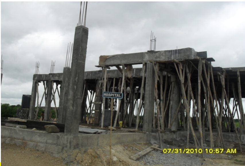
Part GF Slab casted - Hospital building
