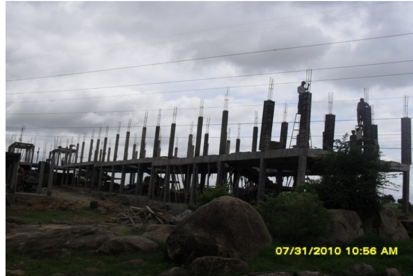
First floor level columns completed - Staff Qtr
