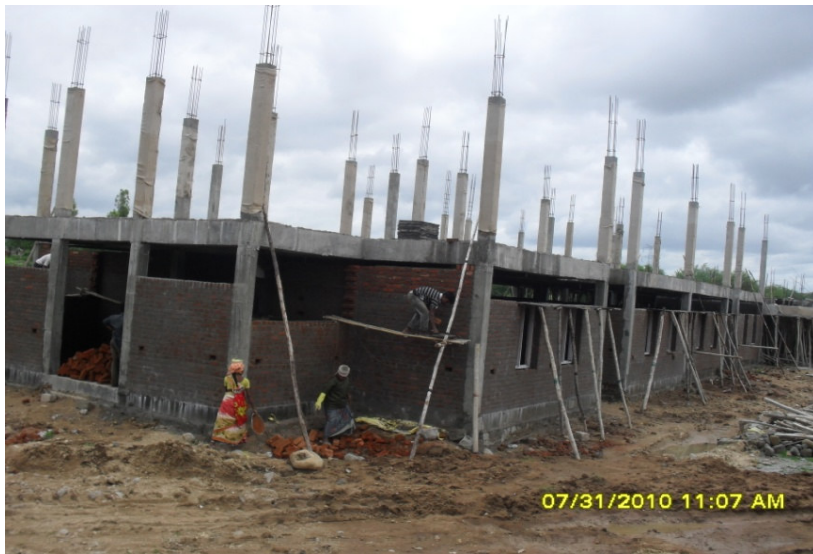
Adults Home- Masonry work in progress
