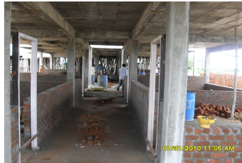
Child.Home - Inside work in progress
