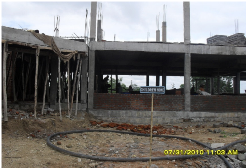
Child.Home - Masonry work in progress
