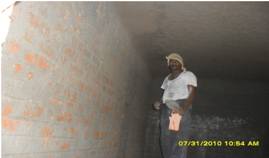
Plastering work in progress at School Building
