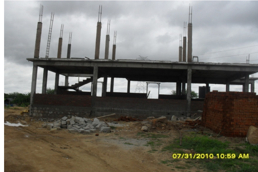
Admin block - Masonry work in progress
