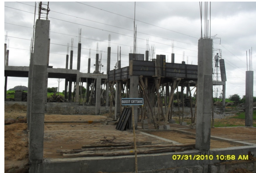
Guest House - Work on progress
