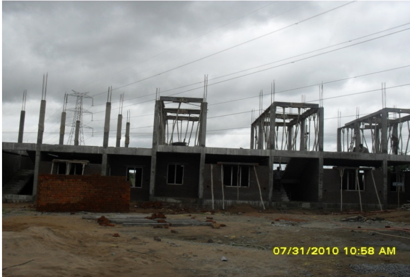
Staff Qtr - FF Shuttering work in progress
