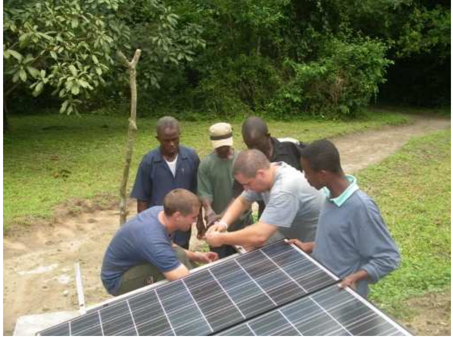
Lahai snr, Paul, Alfred, Simon, Mr Magona and Lahai jnr installing solar panels at Tiwai island. The Tiwai installations doubled as training programs for the installation and maintenance of solar technologies.
