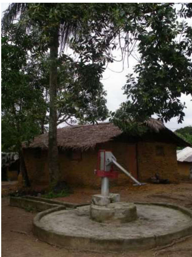
A water-pump installed by EFA at a fresh water well in Perry camp.
