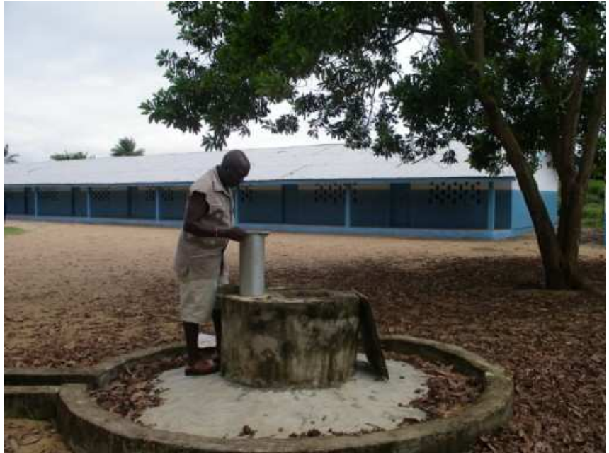
Harry, EFA's Environmental Education Officer, inspecting a well EFA is constructing at a school adjacent to the former Senji camp.
