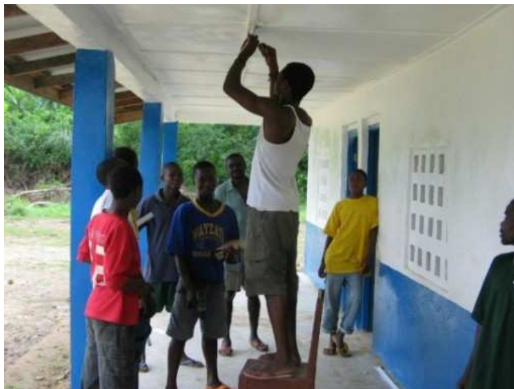
Two-Five, one of the electricians on the project, wiring Tumuquelleh school, Gbarpolu county, in preparation for solar power.
