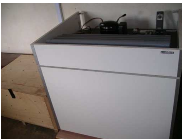
Vaccine fridge and a securely boxed battery-bank. The fridges are powered with independent systems so that they will remain functional even if daily activities and/or poor weather limit the main systems.
