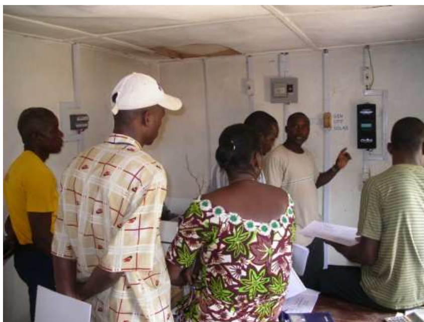
Passing on the knowledge. Freeman Gohu, a volunteer on the project from the University of Liberia, training the staff at Saclepea Community Clinic in the maintenance of their solar power system. The clinic serves a community of 38,000 people.
