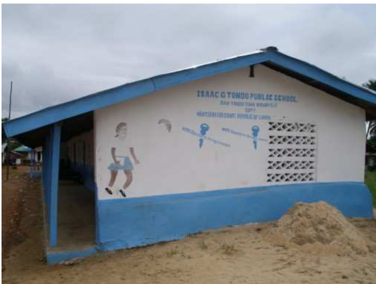
Construction at Isaac Tondo Public School. Beyond our work in environmental education EFA constructs and/or renovated schools in communities with a high population of refugees and/or IDPs.
