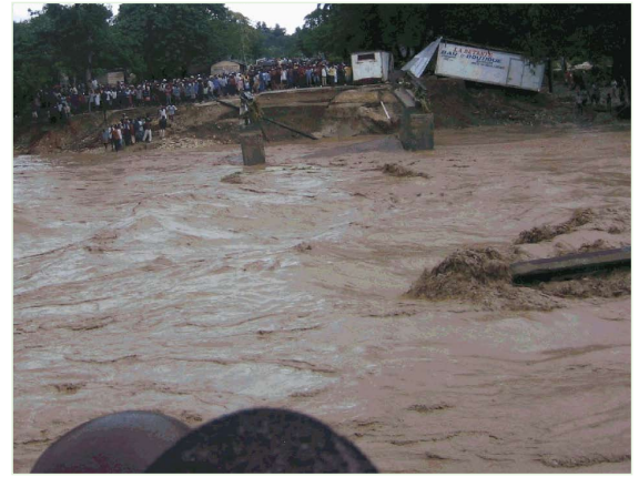
A major bridge collapsed in Mirebalais.
