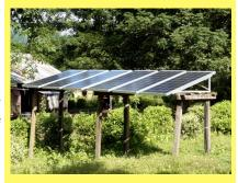
The loads at the facility required (24) 130W solar panels. However, rather than building one large system and distributing the power, we installed (12) 2-panel systems. In the case of the central communications center, many of these systems are in the same room, but we have found that this design leads to much greater reliability and redundancy of equipment where otherwise, the failure of one piece of equipment would shut down the entire operation.
