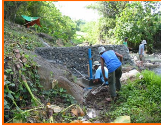
Installed and operational ram pump
