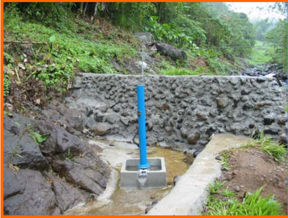
Installed and operational ram pump
