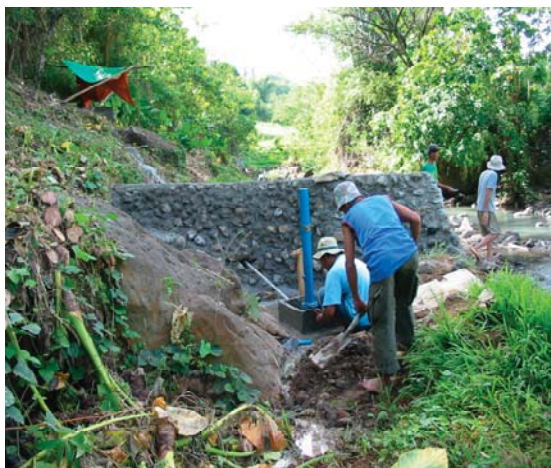
Installing a Ram Pump in Negros
