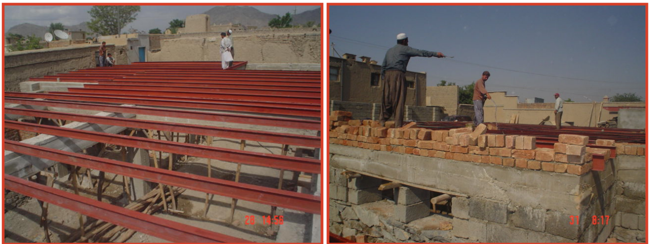
Construction completed of the Ragan Kaman Pre School as of June 2007.
