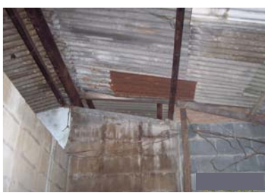
Leaking in the roof
