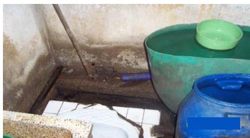
Perpetual flooding in toilet due to low-lying flooring
