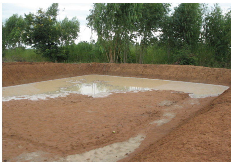
Work of their hands: A finished pond awaiting liming and manuring before water is put in
