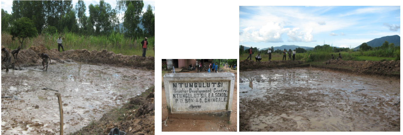
Pond construction at Mtungulusi Primary School
