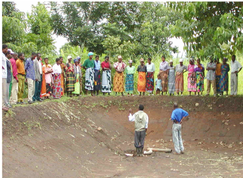
2: Guardians appreciating their good work while a technician helps to fix a water inlet pipe
