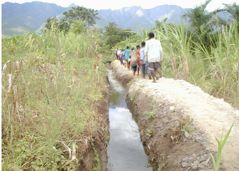
3: Ntanangala canal supplying water to school fish ponds
