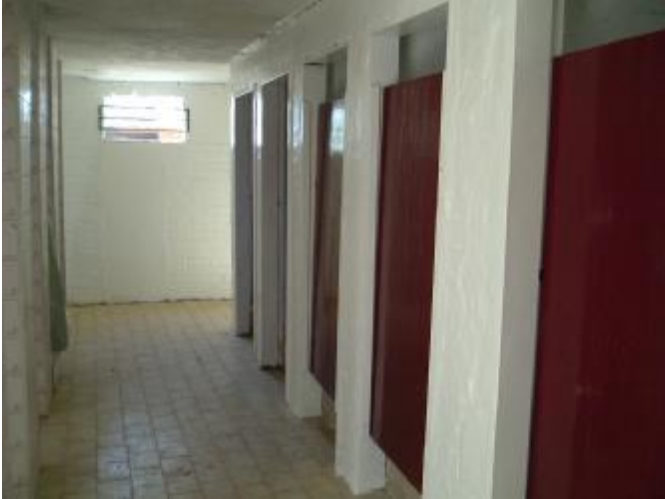
Interior view completed ablution facility May 2007
