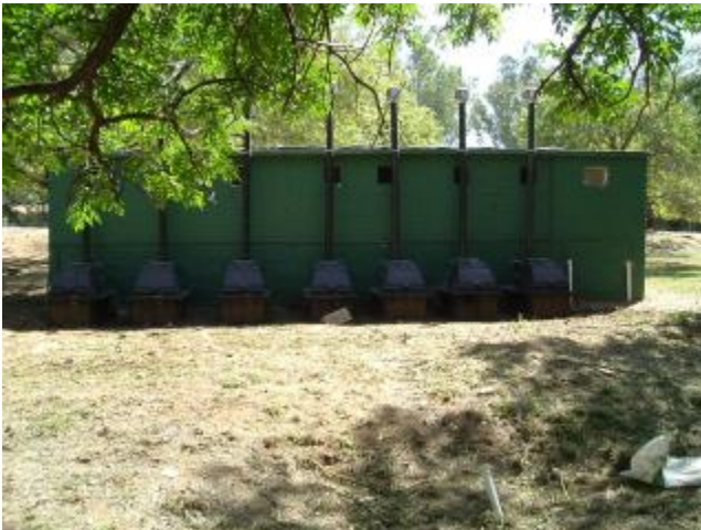
Same building after reconstruction with sanix systems installed May 2007
