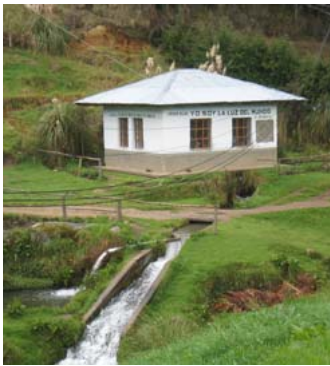
A previously installed hydro power station
