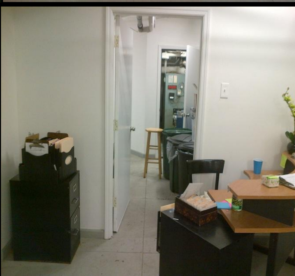
Views of room with furnace before firewall restoration
