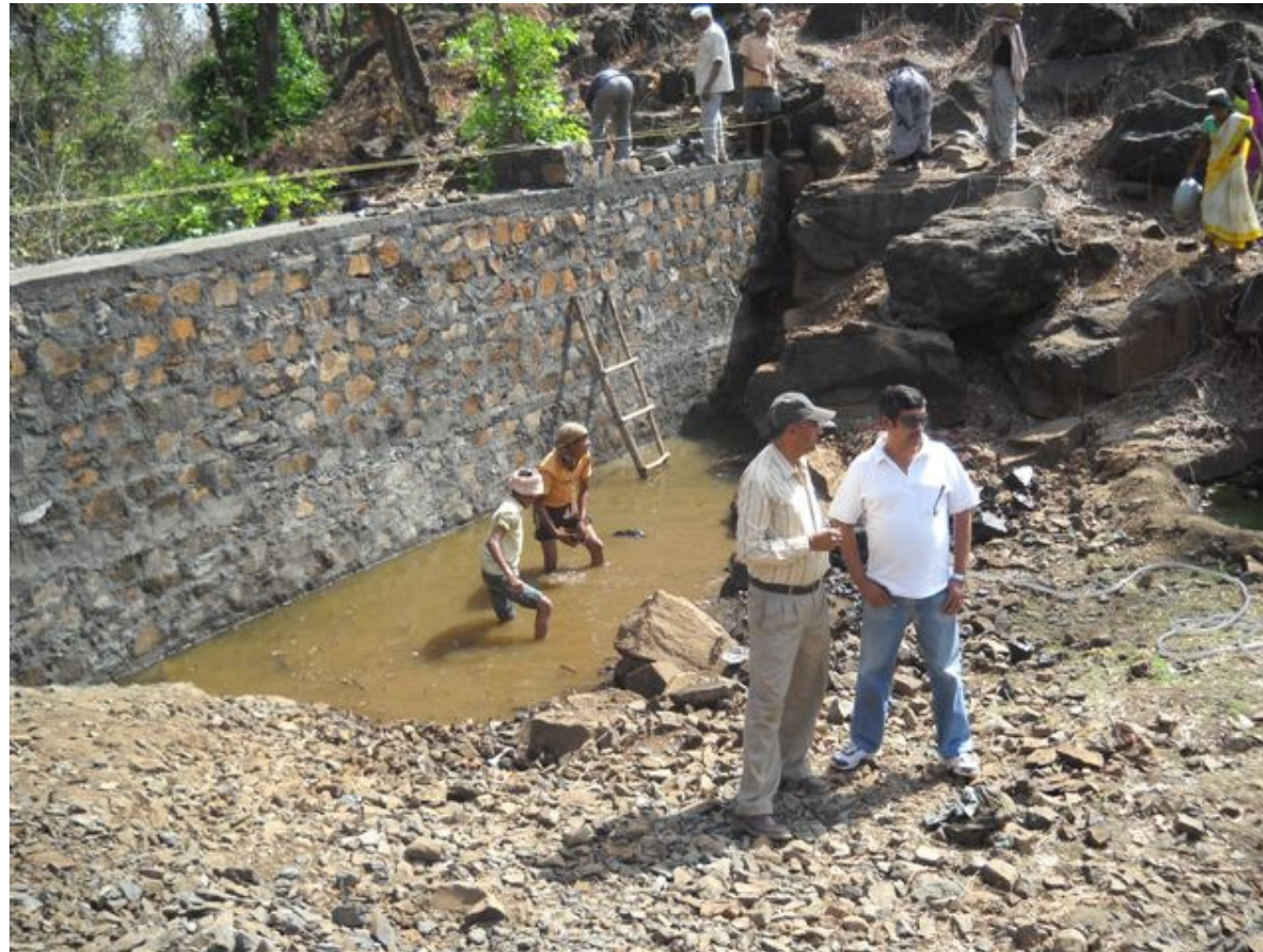
Check Dam Wall at 12 ft. – Raising of Wall Completed
