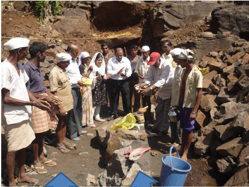
The Foundation for the Check Dam
