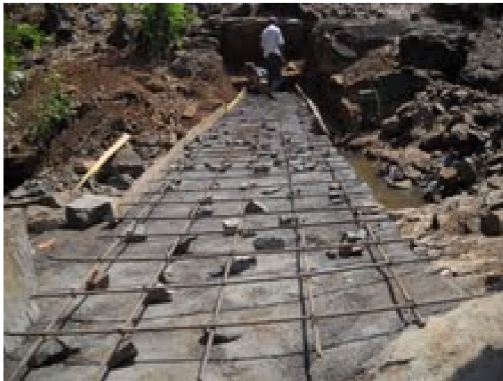
R.C.C. Beam being laid at 4ft. Height, second R.C.C. Beam has been laid at 10ft
