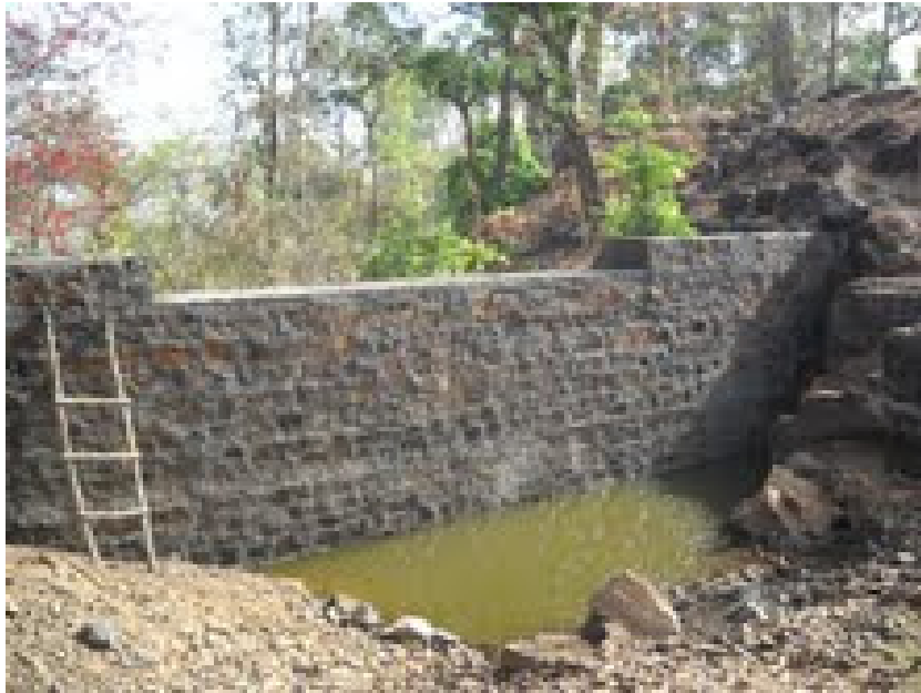
Ends of the wall raised to channelize water flow & allow overflow into Damanganga, Gujarat
