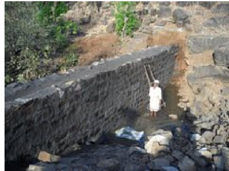
Check Dam Wall at 10ft
