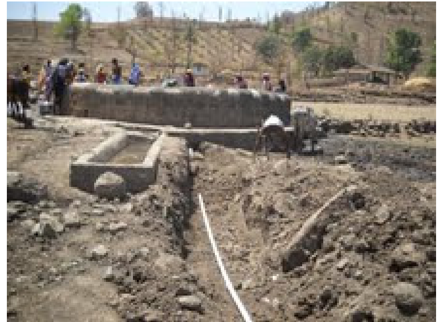
Laying down pipeline from the village well
