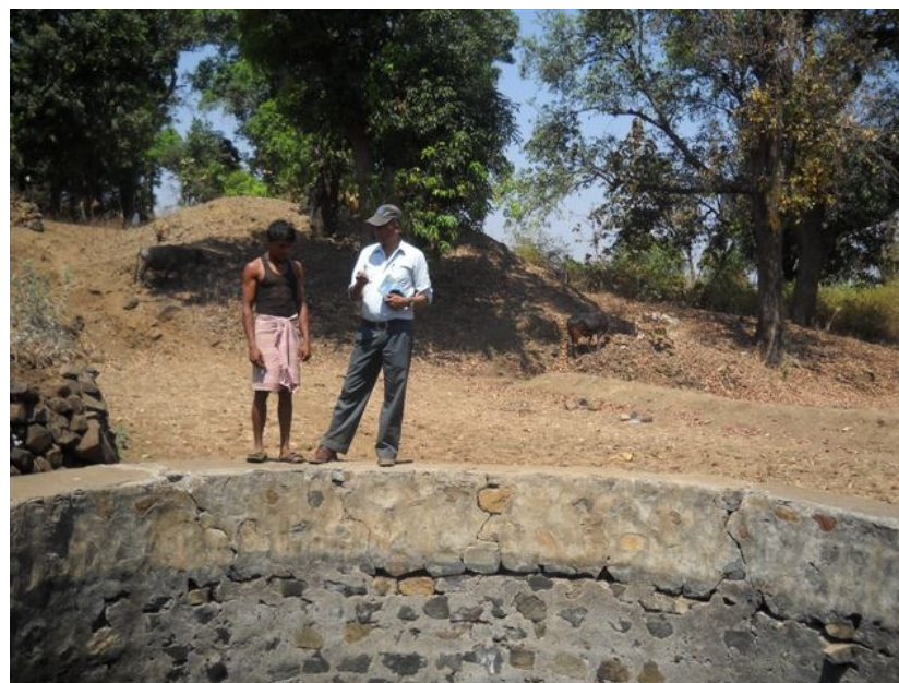
The Vadipada Village Well – in need of repair & cleaning
