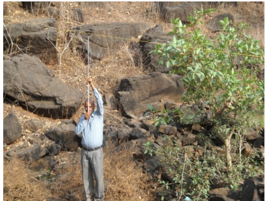
Initial Measurements being taken for Check Dam Construction
