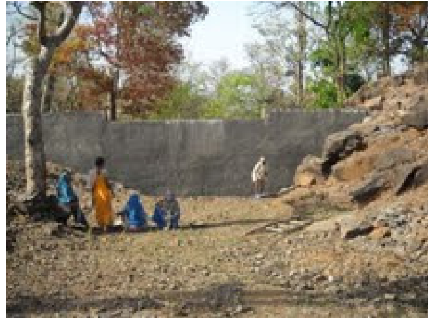
Dam Wall Plastered (65' * 12' * 3')
