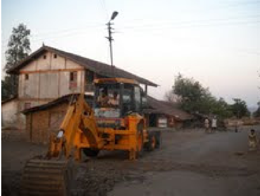
Use of JCB for digging the trench for laying of pipeline beyond the field
