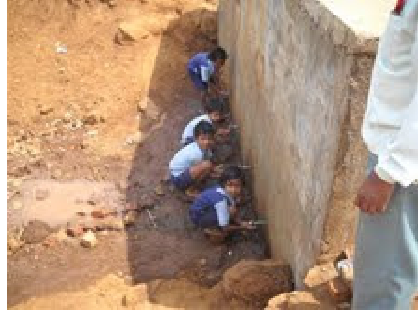
The cement water tank (at the school) which has been connected to the village well
