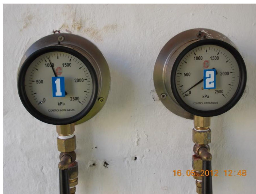
Pressure gauges showing suction and discharge pressures at the Blue Horizon pump station.
