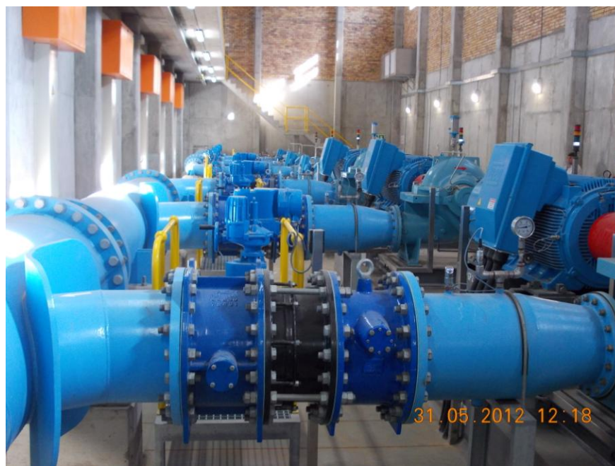
The newly completed Gamtoos booster pump station represents a critical component of the NMBMM's water supply infrastructure.
